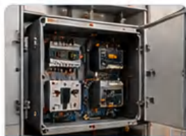
Electrical Enclosures Sealing & Insulation
